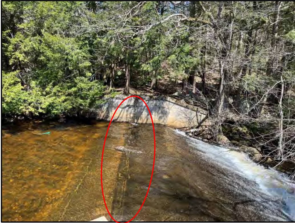
Photo 17 – Spillway and left training wall; note trees on downstream left training wall and flashboard/support slots
