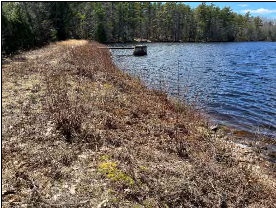
Photo 8 – Upstream slope from left abutment
