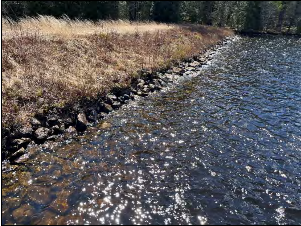
Photo 7 – Upstream slope; note small, rounded riprap extending to just above water line
