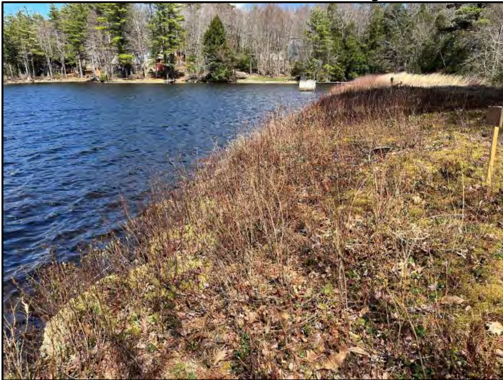
Photo 6 – Upstream slope from right abutment
