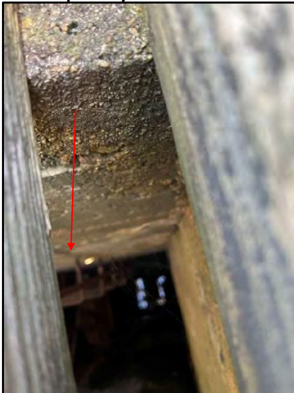
Photo 16 – Interior of the low-level outlet's intake structure; note ladder constructed of bent rebar
