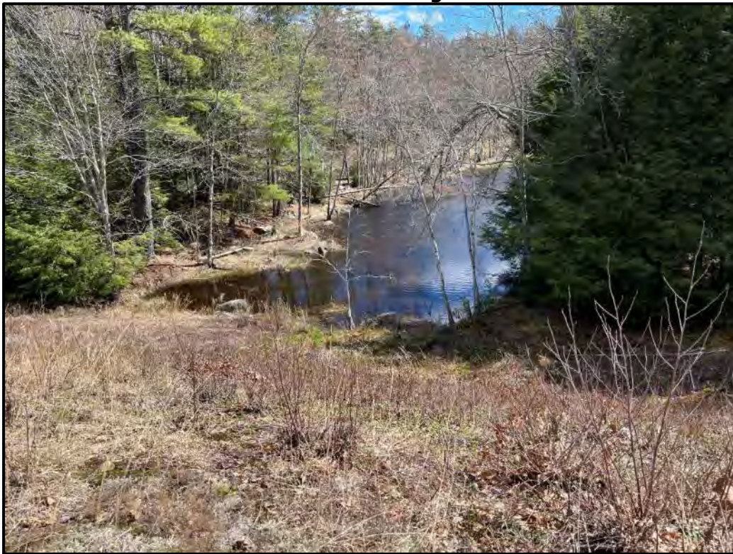
Photo 12 – Overview of tailwater pool at toe of downstream slope
