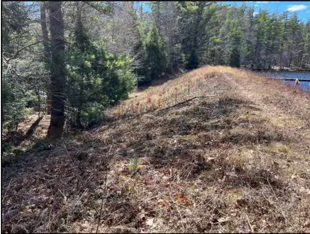
Photo 9 – Crest and downstream slope from spillway; note trees within 20 feet of the dam
